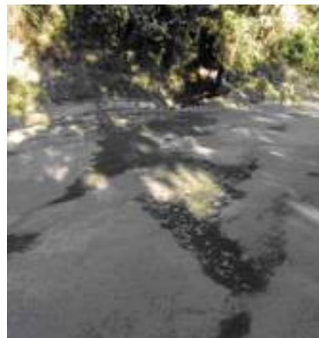
Image 10: Poorly intercepted slope water flowing on roads. signatures of initiation / formation of pot holes.
