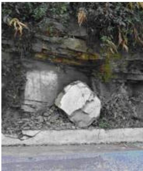
Image 7: Wider spaced intersecting joints forming overhangs that are falling on roads.
