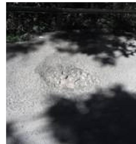
Image 11: Wet roads over a longer period of time showing distress signatures of initiation / formation of pot holes.
